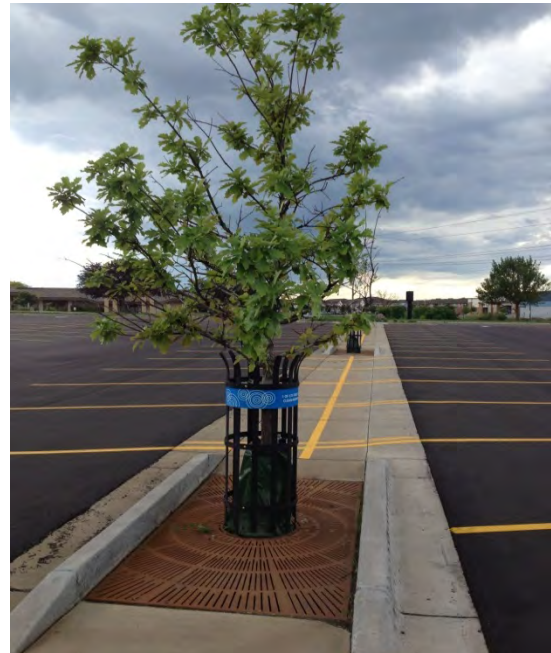
Tree trenches at Maplewood Mall
